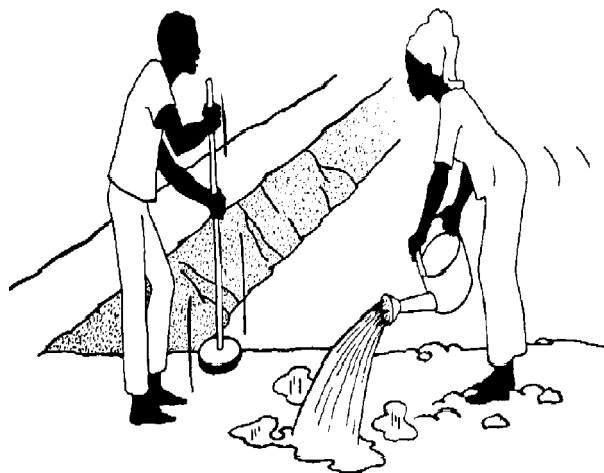
Figure 13: Compacting the dike (Viveen et al., 1985)
