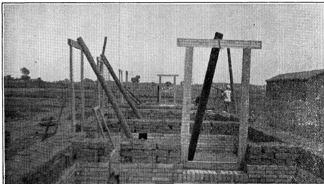
Fig. 90.—Foundation of dwelling, consisting of hard-burned brick; balance of wall to be sun-dried earth brick, seen in Fig. 89.
